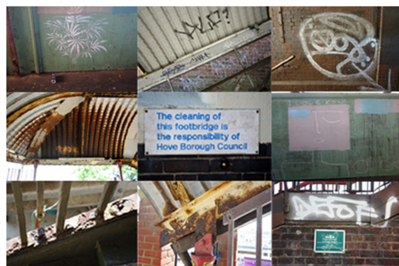
Current Condition of Footbridge
