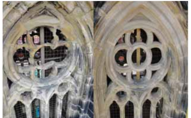
Pre & Post repairs – NE Tower
