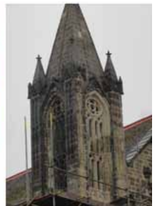
Re-pointing and the SE Tower
