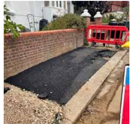
A recently removed elm stump and potential tree pit asphalted over at the junction of Chanctonbury and Highdown Road
